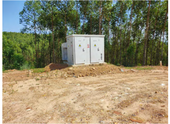
风力发电场区箱变现状
